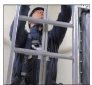
**Step 3 –** With a solid body position technician 1 grabs the hanging safety wire with gloved hands. Then holds tight on the safety wire and performs a fast hard lateral heave towards his/her body.
