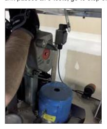
**Step 5 –** If locked, reset the BlocStop to ensure the jaws are open by pulling downward on the reset lever. Move up the cabin lift 0,5 mts above the landing platform by pressing the up button on the pendant control.
